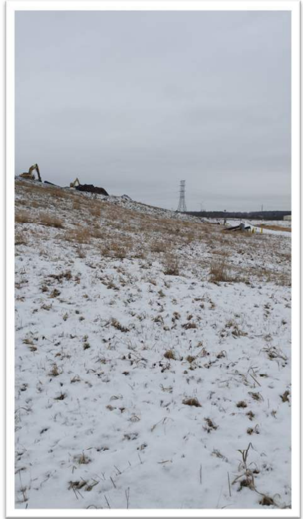
56. N Corner Outer Slope Top of Slope Facing SW
