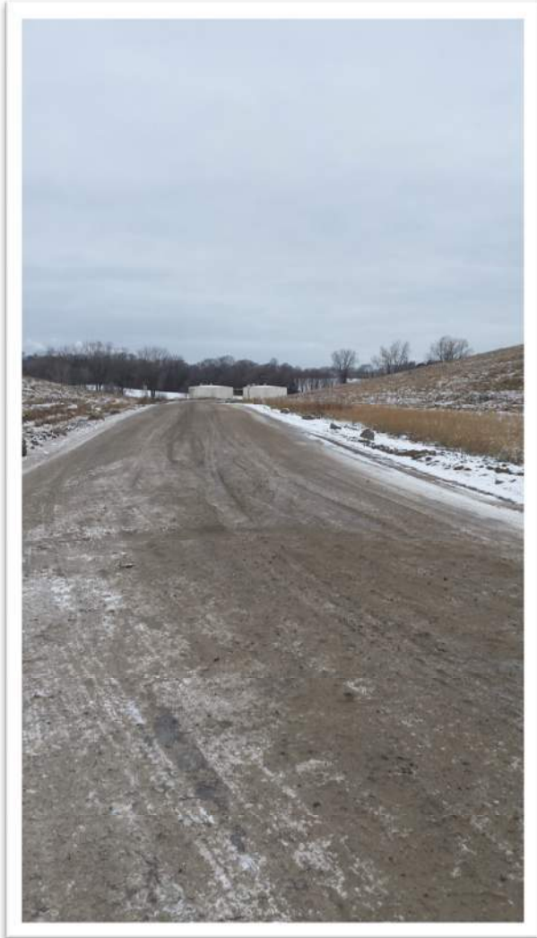
11. WSW Interior Slope Middle of Slope Facing NW
