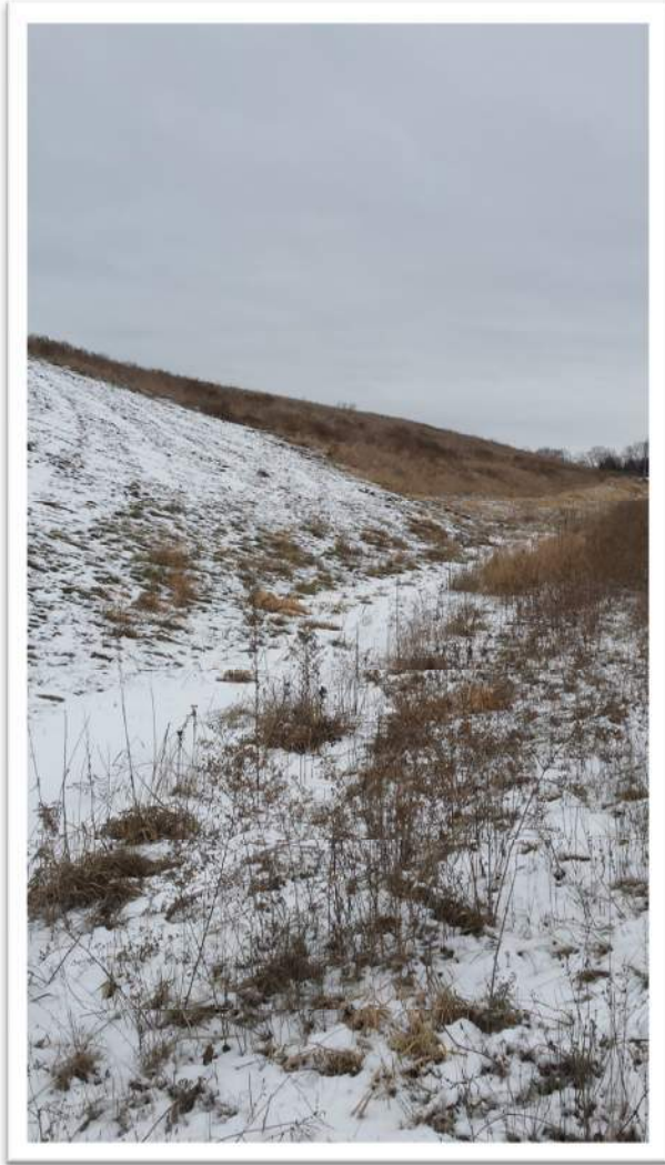
49. SE Outer Slope Top of Slope Facing NE
