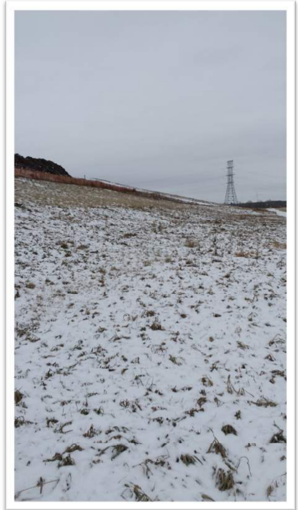
58. NW Outer Slope Bottom of Slope Facing SW
