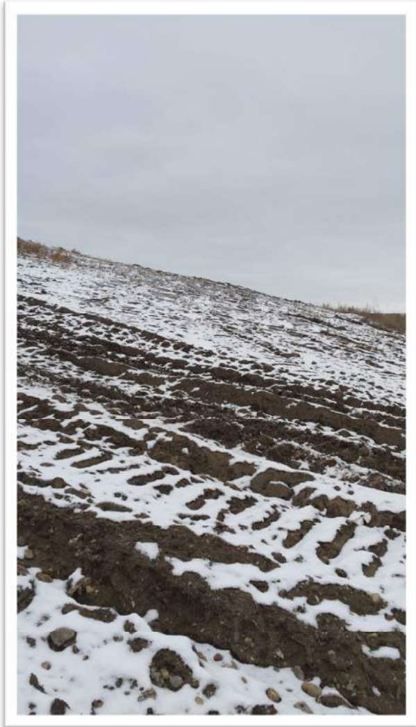
45. SE Outer Slope Top of Slope Facing NE
