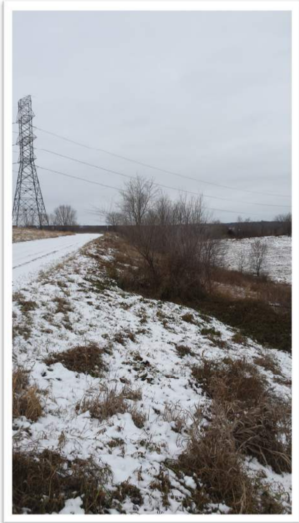
15. W Corner Outer Slope Bottom of Slope Facing SW
