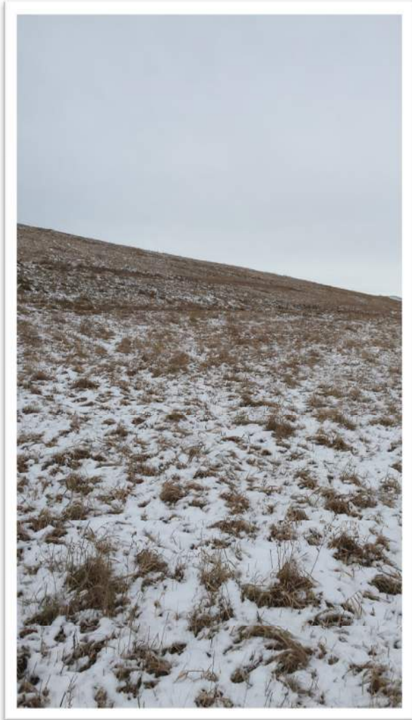
19. SW Outer Slope Top of Slope Facing SE
