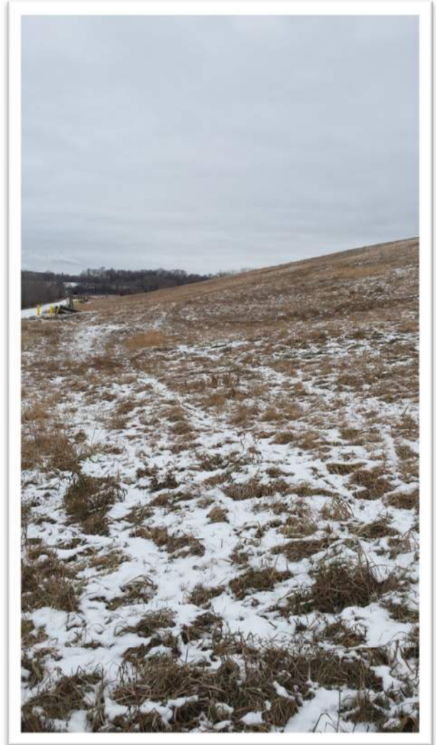
28. SW Outer Slope Top of Slope Facing NW
