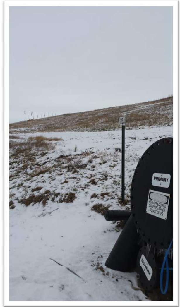
54. NE Outer Slope Top of Slope Facing SE
