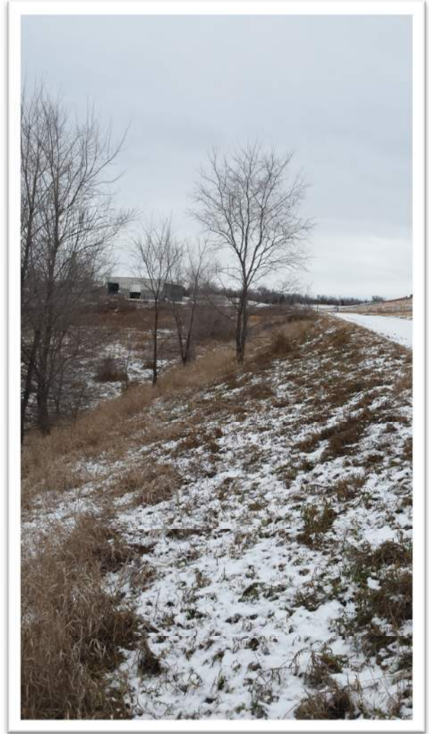
18. W Corner Outer Slope Bottom of Slope Facing NE
