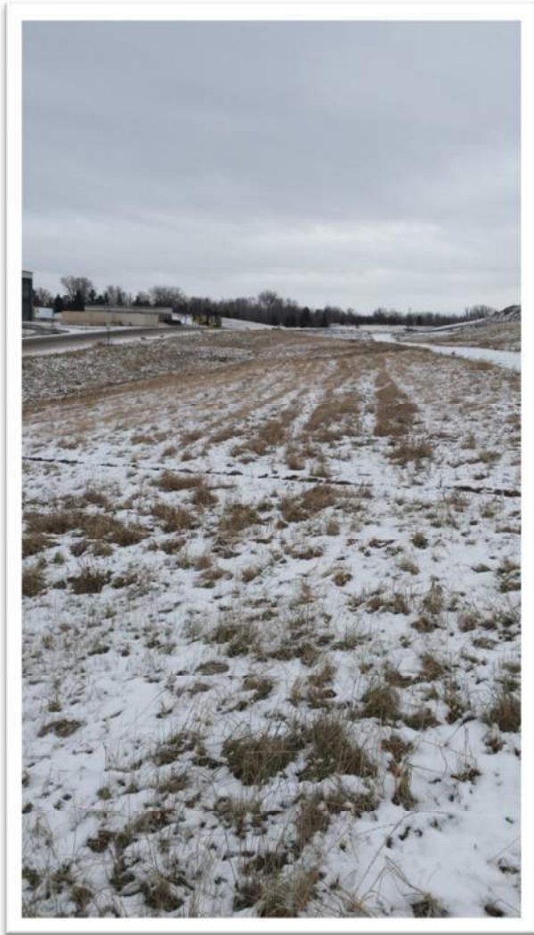
1. NW Outer Slope Bottom of Slope Facing NE
